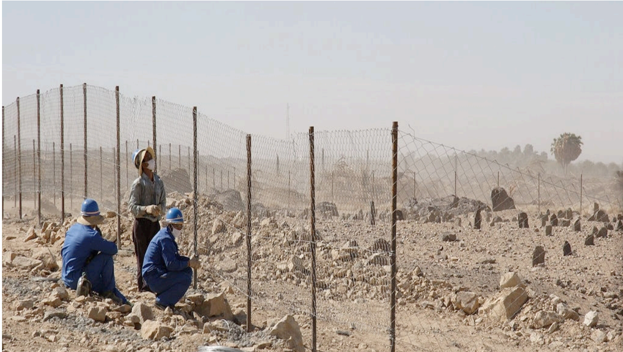
Chinese workers at a construction site in Africa (David Haberlah)
